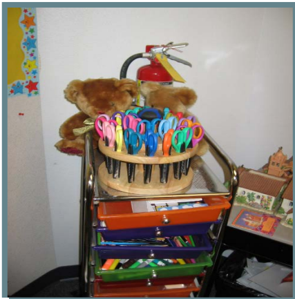
Fire Extinguishers Can't Be Used if They Are Blocked
